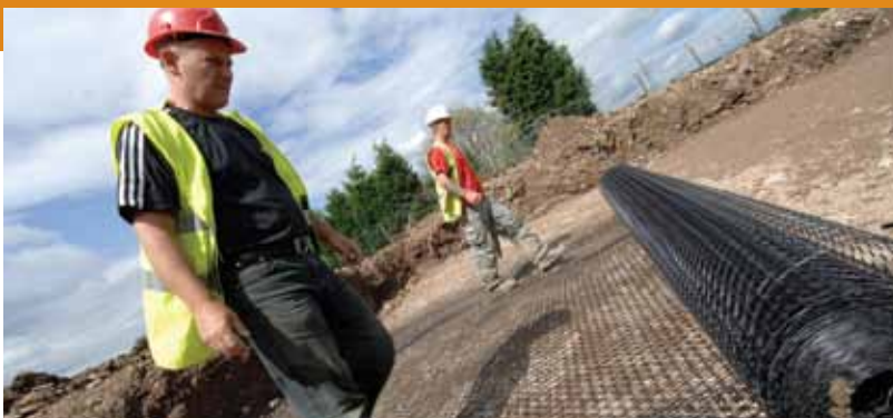
TriAx installation, Stoke
