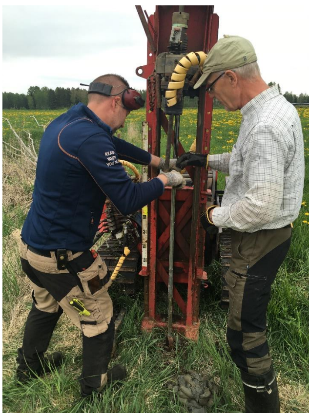
Figure 13. Drilling of groundwater tube, Ämnäsviken field, 2019.
